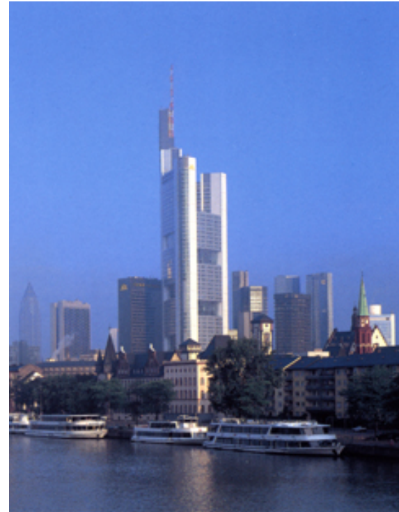
Commerzbank Frankfurt am Main, 1997 Foster Associates
