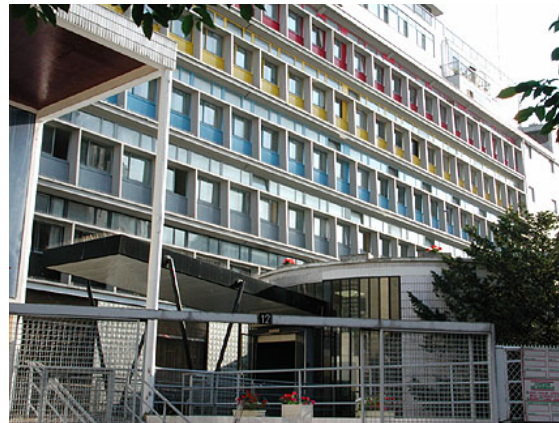
Modified with brise soleil added
